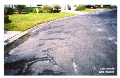
is the interpretation of symmetrical cracking. If your community has a soil-cement base, also known as a floating base, and they are trying to get rid of the symmetrical cracking on the property, give it up! You will soon find within a year or two of a new overlay that the exact same cracking, which you just covered up, will return in the exact same pattern that was there before. This is
